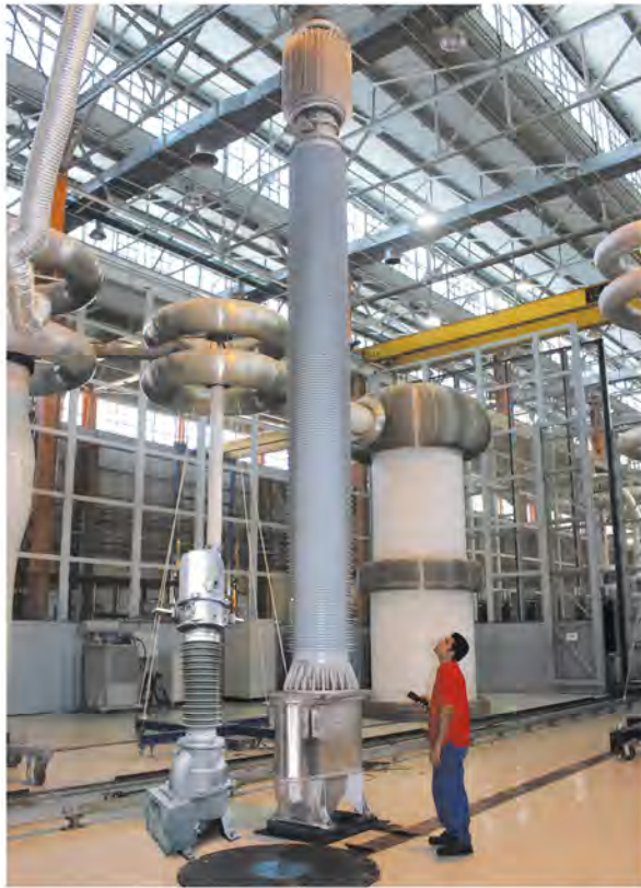
Tank Type Current Transformer (IMB) 72.5 - 800 kV
